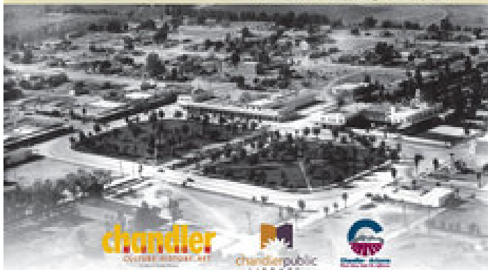
Aerial view of Chandler, looking southwest, c. 1932
