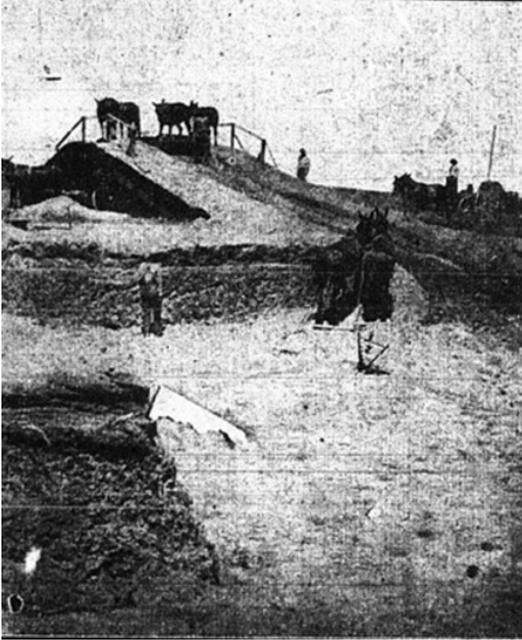
In the image above, a team of mules pulls dirt up a small incline on the San Marcos site using a Fresno Scraper.
